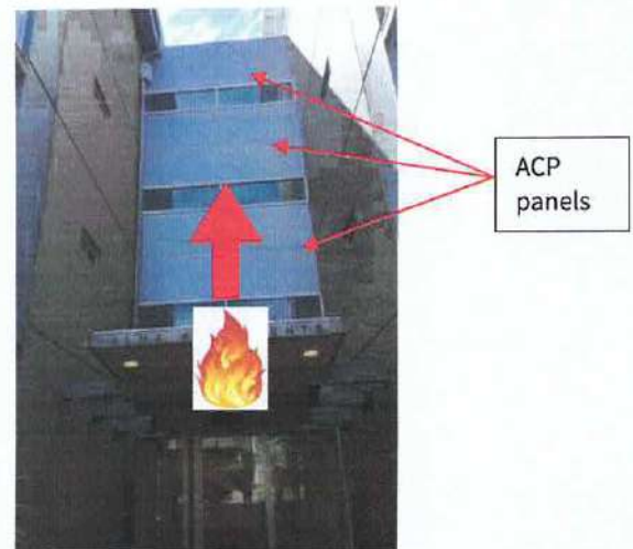
Figure 4.3 – Fire Scenario 2 – External Façade
